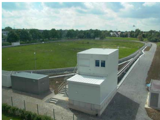
Fig. 1: Test track with control and substations
